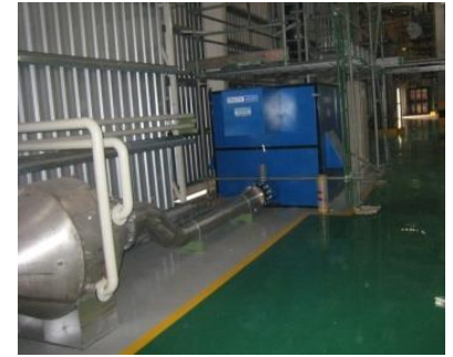
Roots blower package with air cooler set
