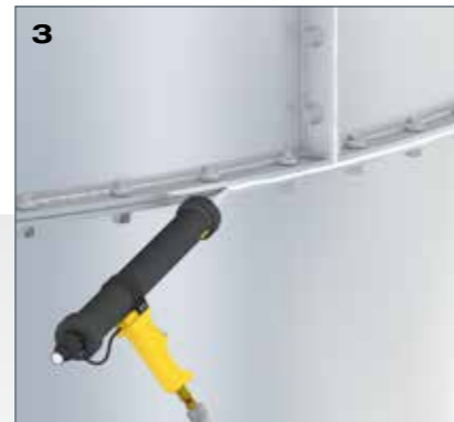
3 Seal the flanges on the outside.
