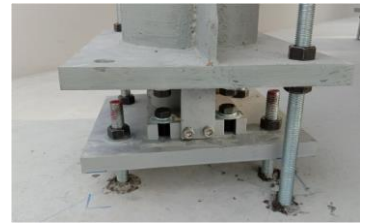
PVC Silo & DOA Storage tanks /weight monitoring system
