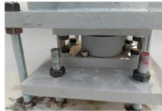
PVC Silo & DOA Storage tanks /weight monitoring system
