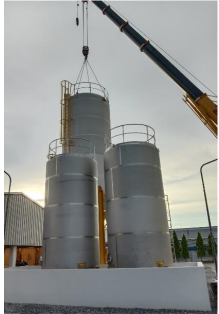
Stainless steel 304 DOA Storage Tank, Size 34 m 3
