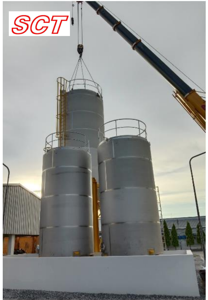
Stainless steel 304 DOA Storage Tank, Size 34 m 3
