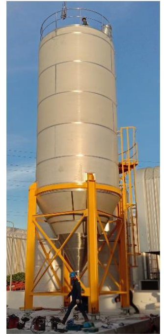
Stainless steel 304 PVC Resin Silo, Size 100 m 3
